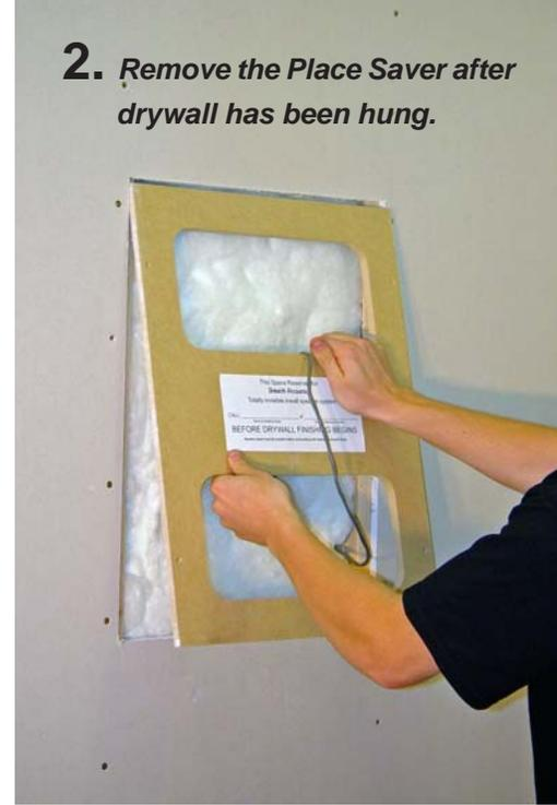
This area is to be used for feathering out the joint compound onto the wall providing a smooth transition from the speaker panel to the wall.
