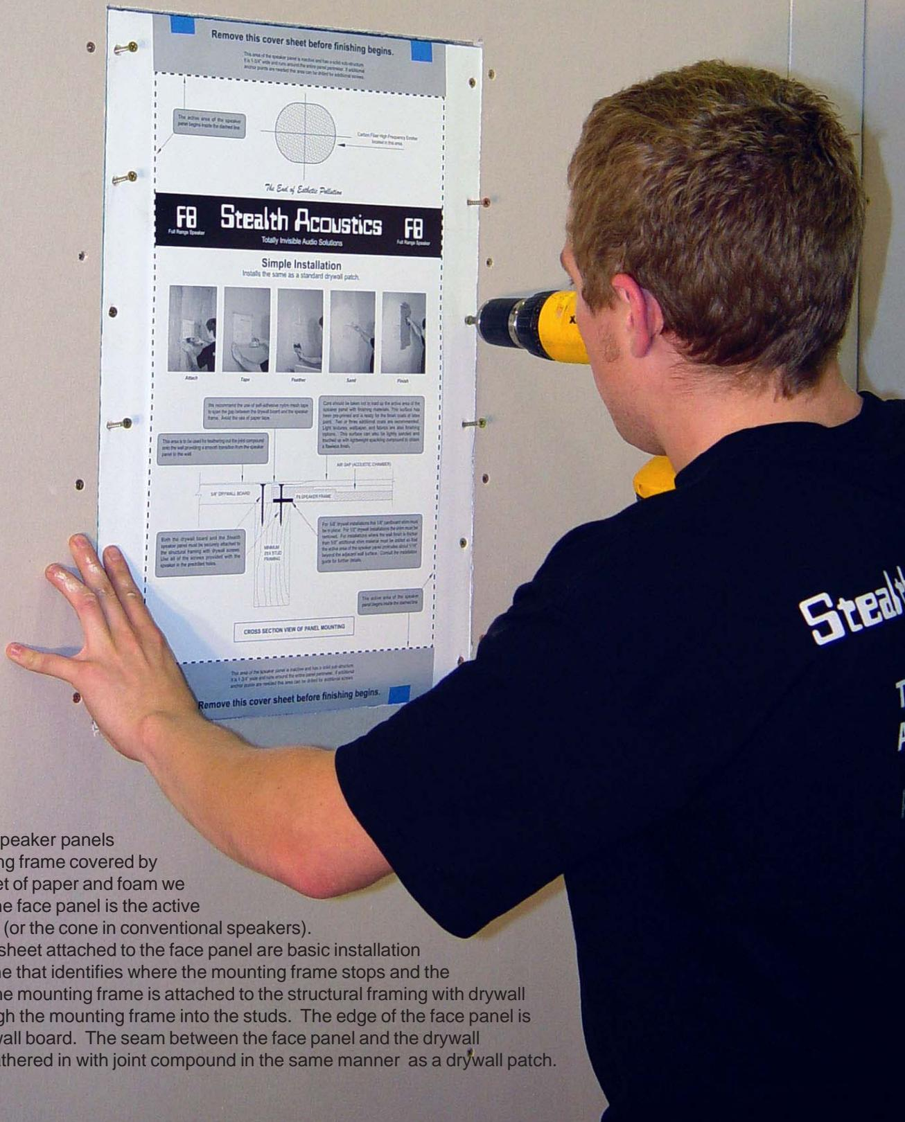
All Stealth Acoustics speaker panels are built with a mounting frame covered by a 3/16" multilayer sheet of paper and foam we call the face panel. The face panel is the active surface of the speaker (or the cone in conventional speakers).
